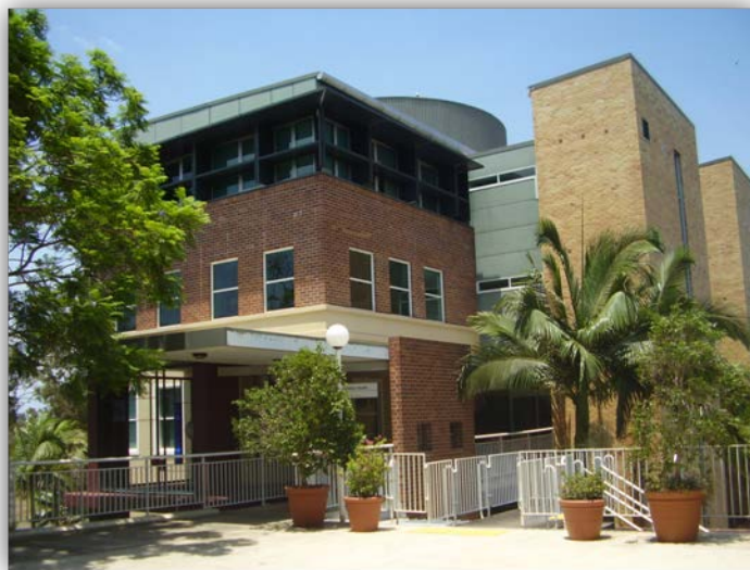
The Public Health Building, Herston
